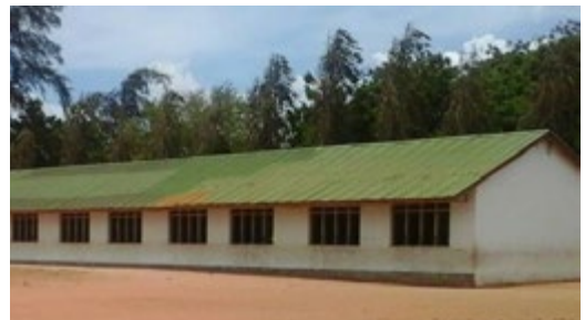
Students and teachers at Boyani Primary school receiving desks; and the 15 classrooms constructed at Marereni Primary School by Krystalline Salt Ltd. (Photo: Courtesy)
